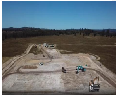
Ledonne Construction of the Bundarra Sewerage Treatment Plant in February 2021. equipment.
